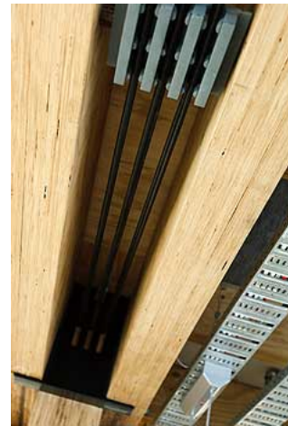
Tensioning cables are an innovative feature of the building's seismic engineering
