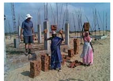
Foundations before brick work
