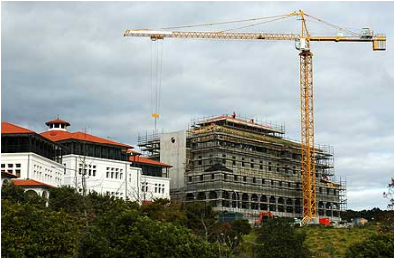
View of the new library extension under construction.
