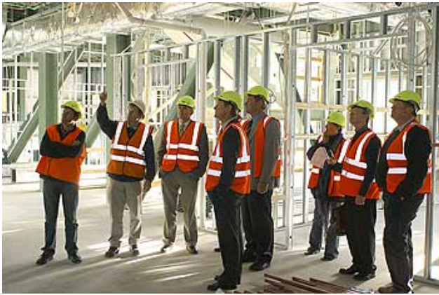
Members of the Hopkirk Foundation inspect construction of the new facility
